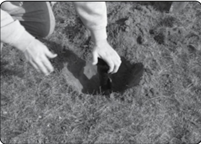
Line up Speedy Sleeve with the top of pipe and slip it over the pipe. Then push the sleeve down over the pipe by hand as far as it will go.
