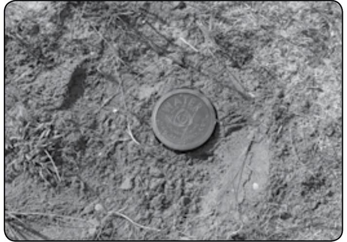
Fill in the hole around the curb box and compact the area flush with existing grade.
