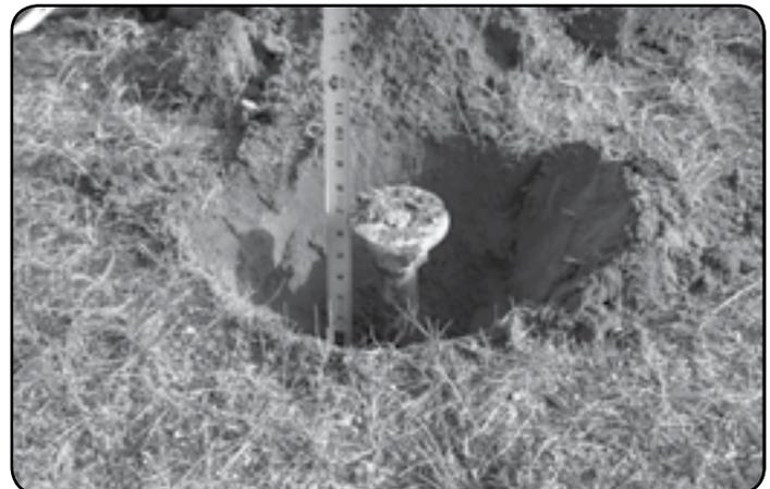
Using a tape measure, verify the distance from the grade to the top of the pipe. The minimum dimension is 1" below the grade, which allows for a flush installation; the maximum is 15".
