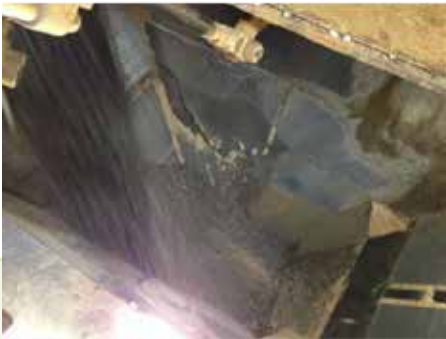
Photo of the internal sides of the hopper, showing the worn and uneven surface.
