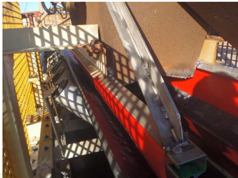
Below: Close-up image of conveyor chute and Snap-Loc after installation.
