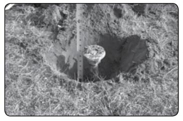
Using a tape measure, verify the distance from the grade to the top of the pipe. The minimum dimension is 1" below the grade, which allows for a flush installation; the maximum is 15".
