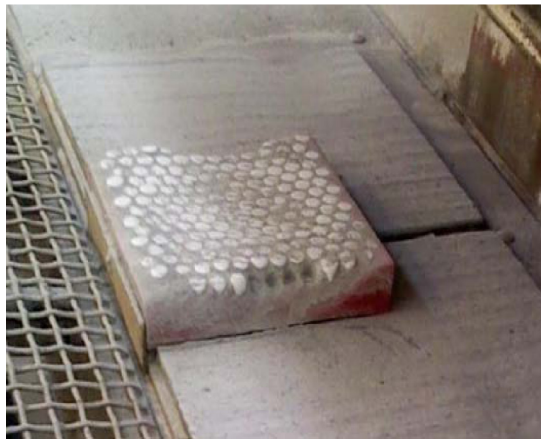
Photo taken on site at Leslie Vale Quarry 15 months after installation
