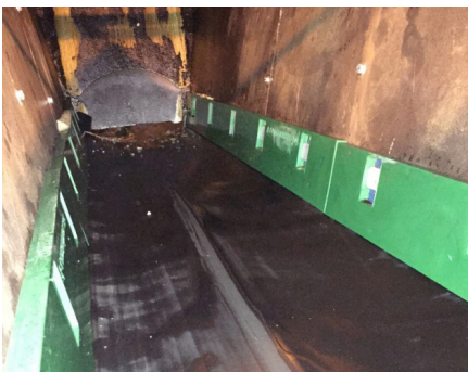
Above: Photo of the Load Zone Containment Skirting installed.
