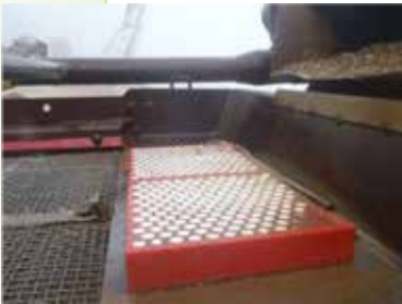
2011 photo of Redi-Liner ceramic in place after 6.5 months
