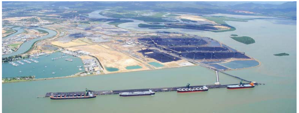
The Port of Gladstone is Queensland's largest multi-commodity port, housing the world's fourth largest coal export terminal and covers an area of 4321 hectares of land.
