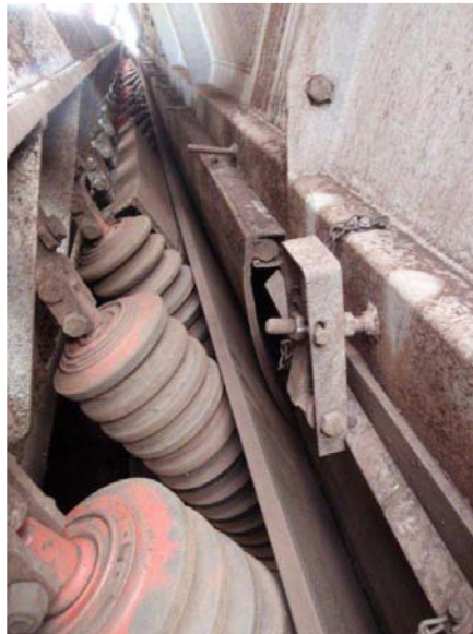
Photo taken February 2013 of Snap-Loc Dust Seal System in place on slider beds at the Power Station, Traralgon, Victoria
