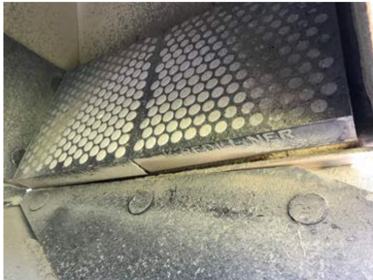
Redi-Liner Ceramic panels installed
